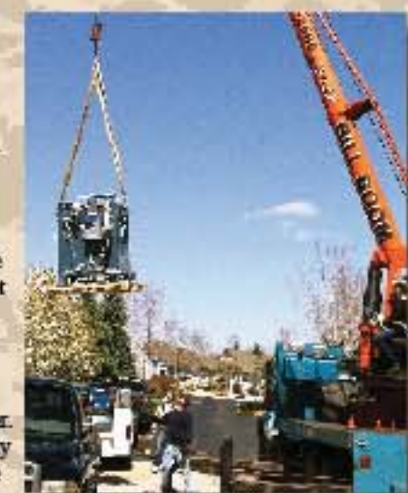
Spare Boiler is lifted from the delivery truck into our building
